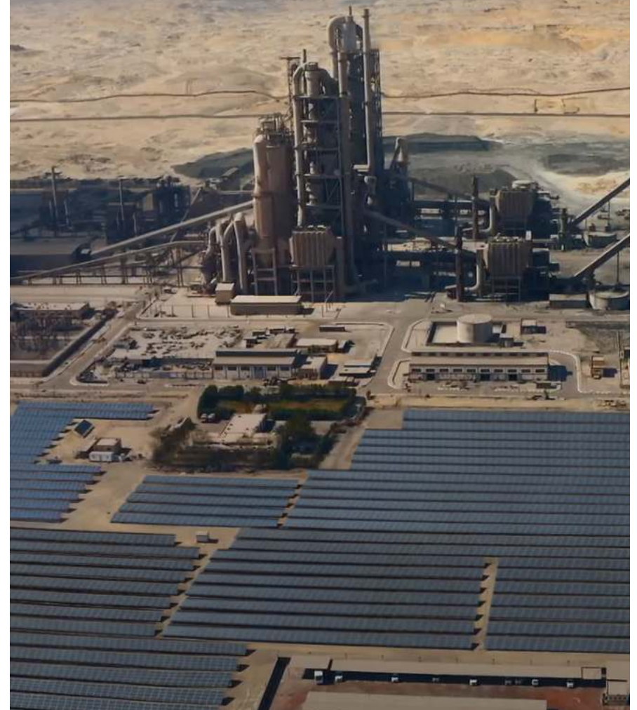
ACC SOLAR PANELS IN PLANT
